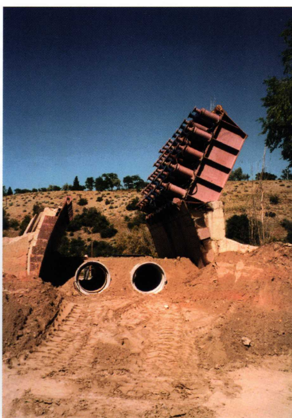
The soil cell at Utah State University was used to test the strength of the Danby liner process.
