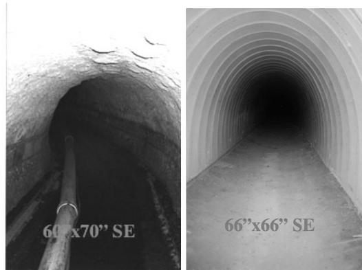
**Figure 1.** Semi Elliptical Sewers in Los Angeles.
