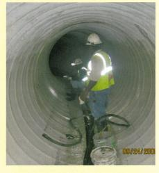
Material Design). The grout consists of Portland cement (57 percent), Fly Ash (43 percent), and water and super-plasticizer admixture. Although the design is based on a grout compressive strength of 6,000 psi, typically the tested 28-day strength is 7,000 – 9,000 psi. The grout will normally set-up in four to 5 hours (firm to the touch) and develop a compressive strength of more than 1,000 psi in 24 hours.
