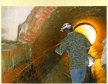
plug also served to prevent short-circuiting of the ventilation system. Even during dry weather there was a small base flow in the storm sewer. A small sand bag weir and submersible pump was installed at the upstream manhole which was piped to discharge at the downstream manhole.
