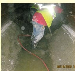
the injection point. The grout is very fluid (18 – 25 second standard flow cone).
