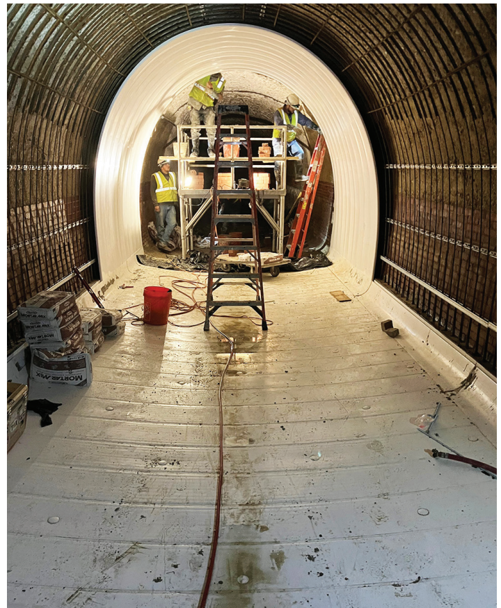
Composite solution, rebar and start of the Danby liner; grout was later installed in-between.
